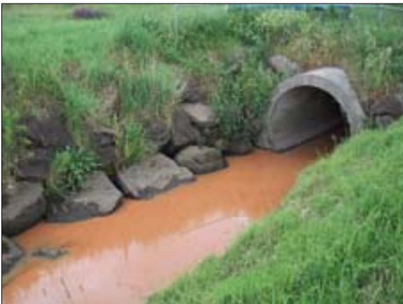
Discolouration in a Darebin Creek stormwater outlet is an example of point source pollution.
